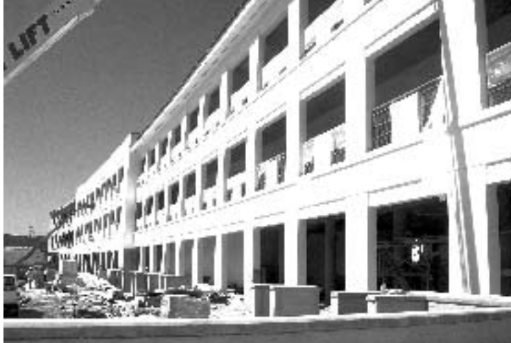
The new three story building located behind the main building
